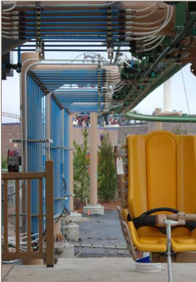
Screw type beam clamps
